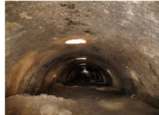
Inside one of the tanks
