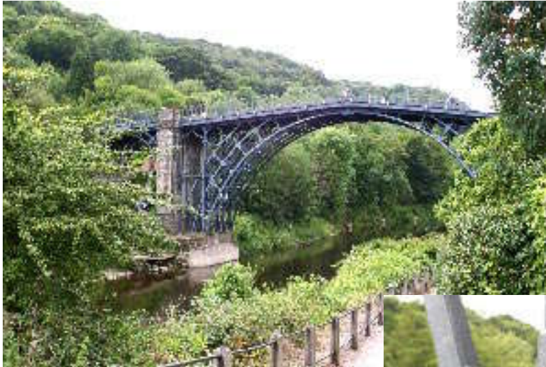
The bridge across the Severn Gorge built in 1779 out of cast iron smelted with coke
